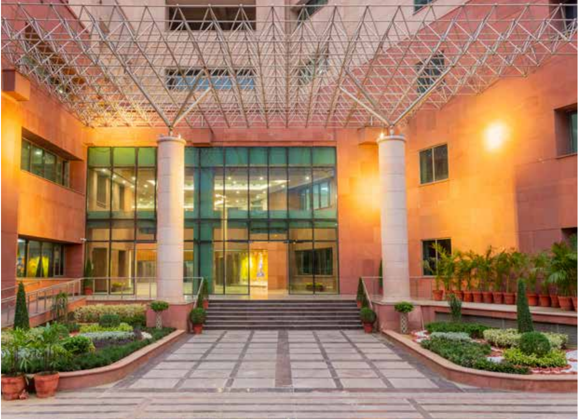
Entrance Gate, Additional Building Complex, Supreme Court of India
