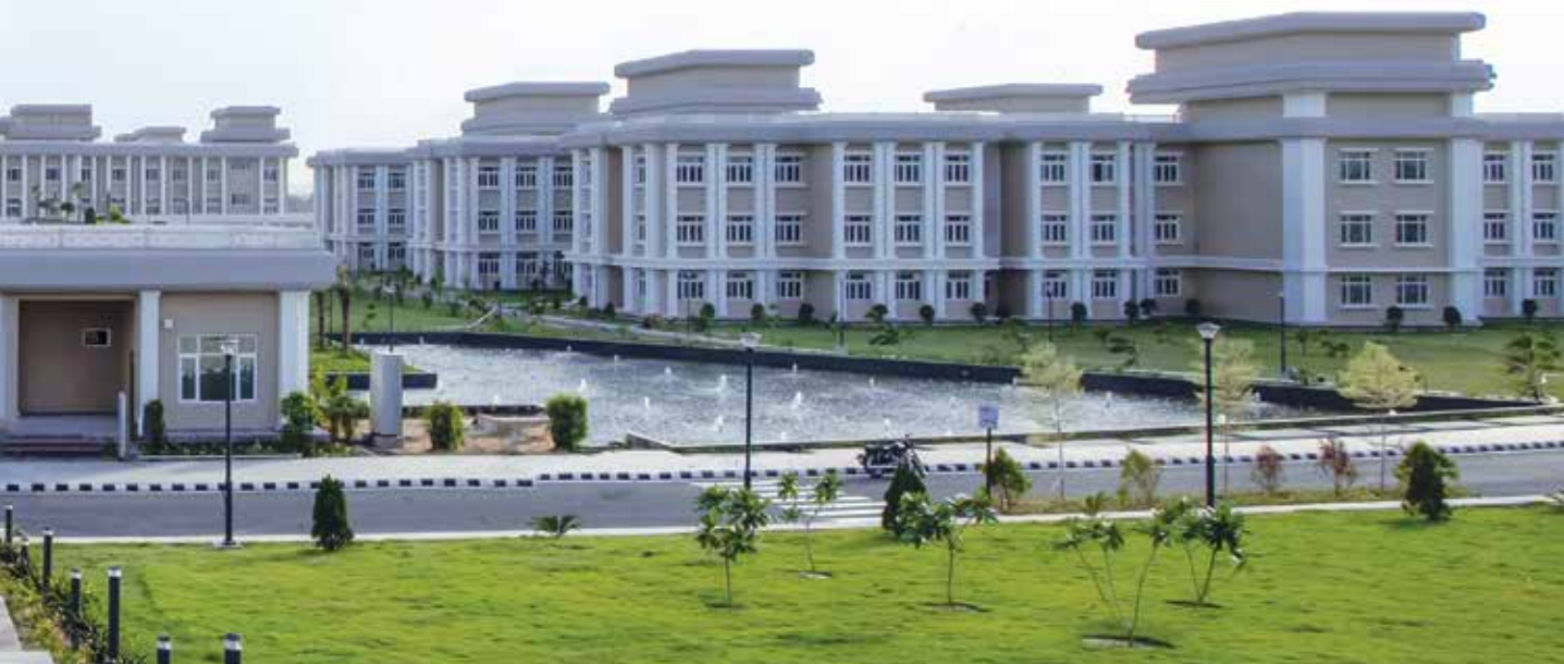
New Building of the High Court at Ranchi
