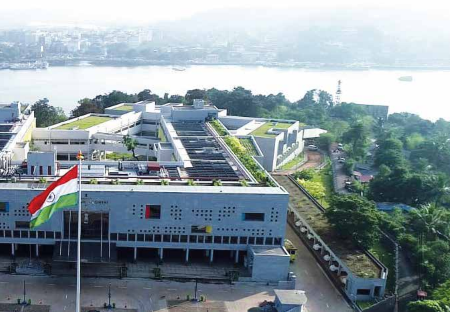
Aerial view of the Seat of the Bombay High Court at Goa
