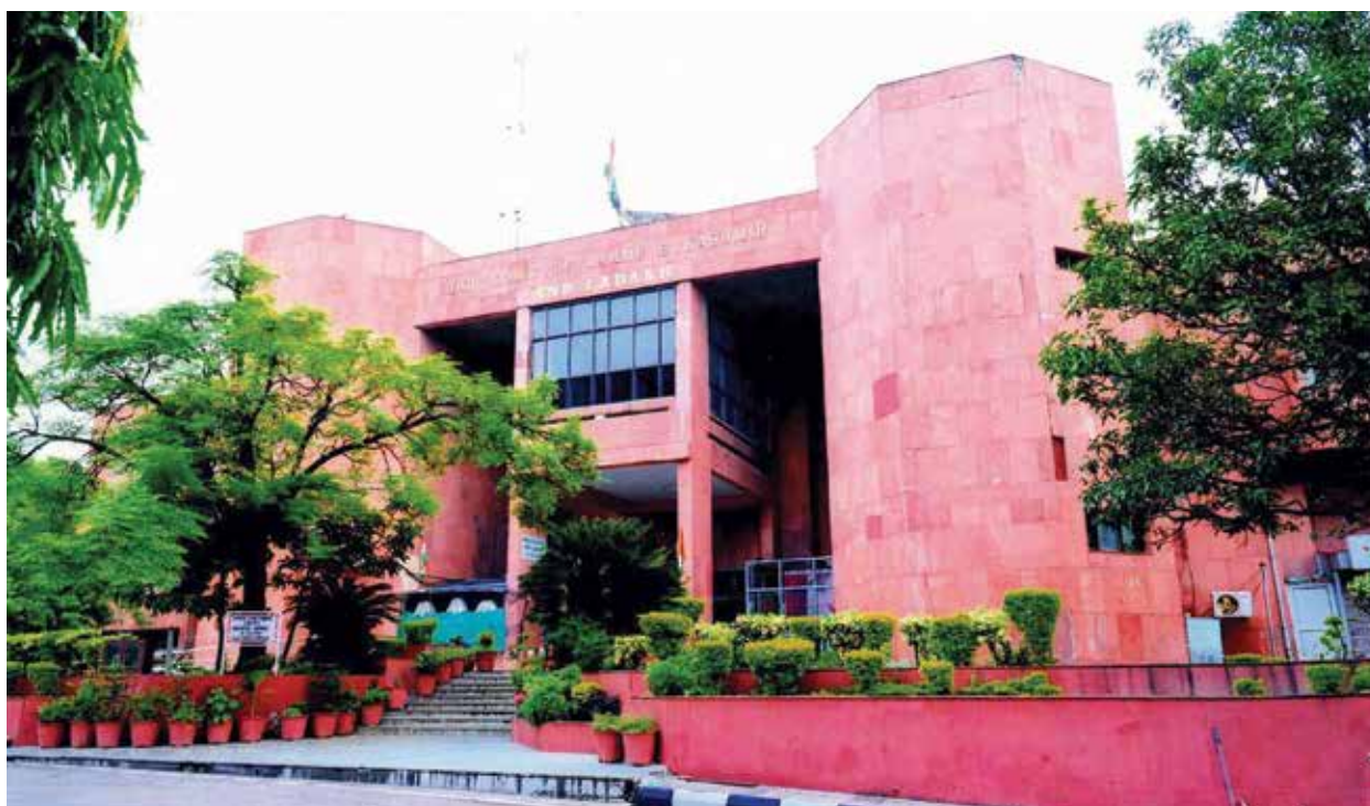
High Court Building at Jammu
