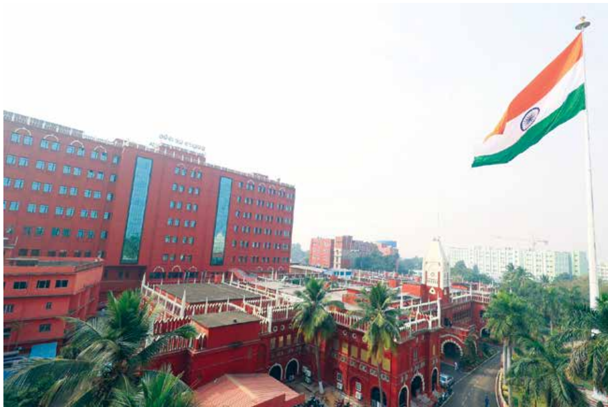
Aerial view of the High Court
