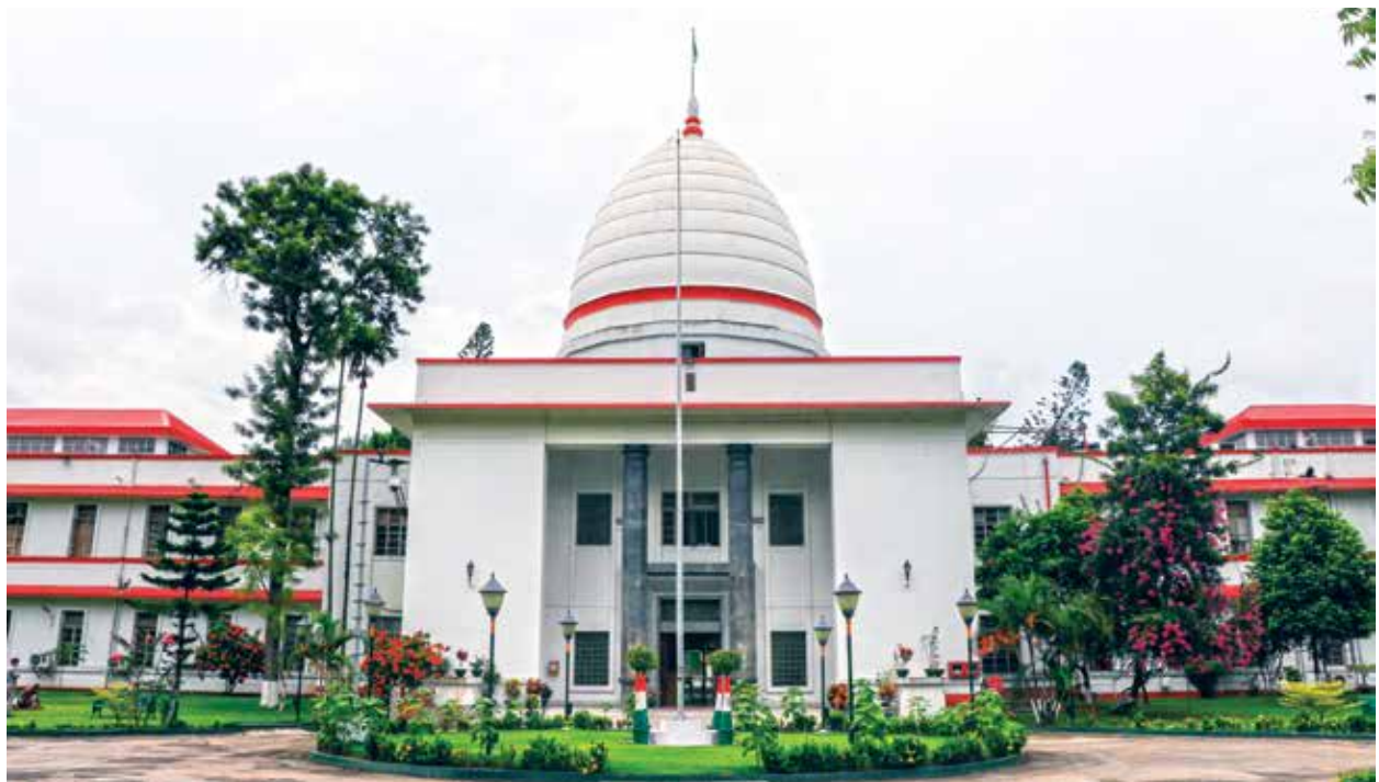
Old High Court Building at Guwahati
