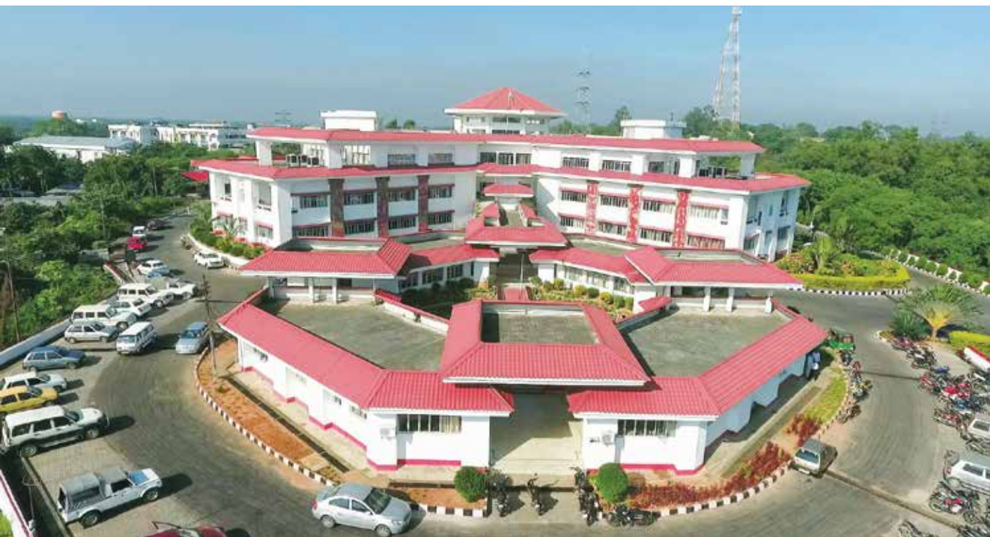
Aerial view of the High Court
