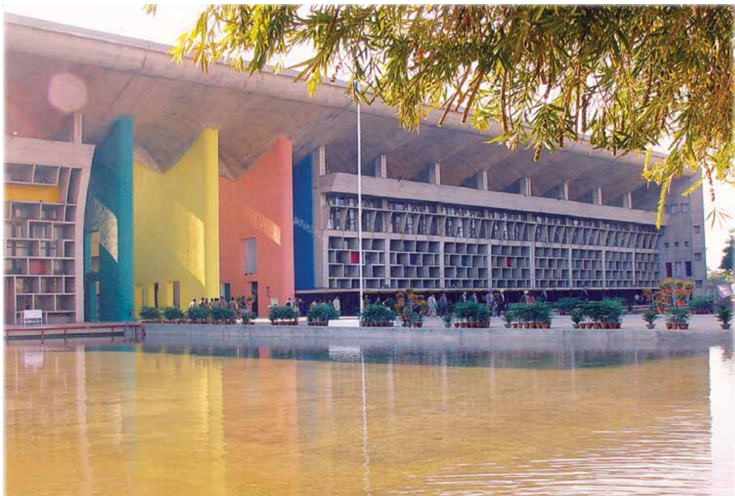
Main Building of the High Court
