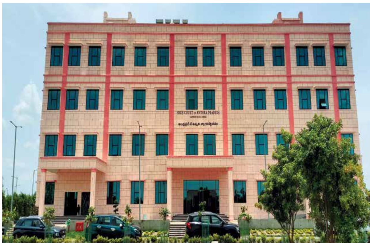
Front view of the Annexe Building of the High Court
