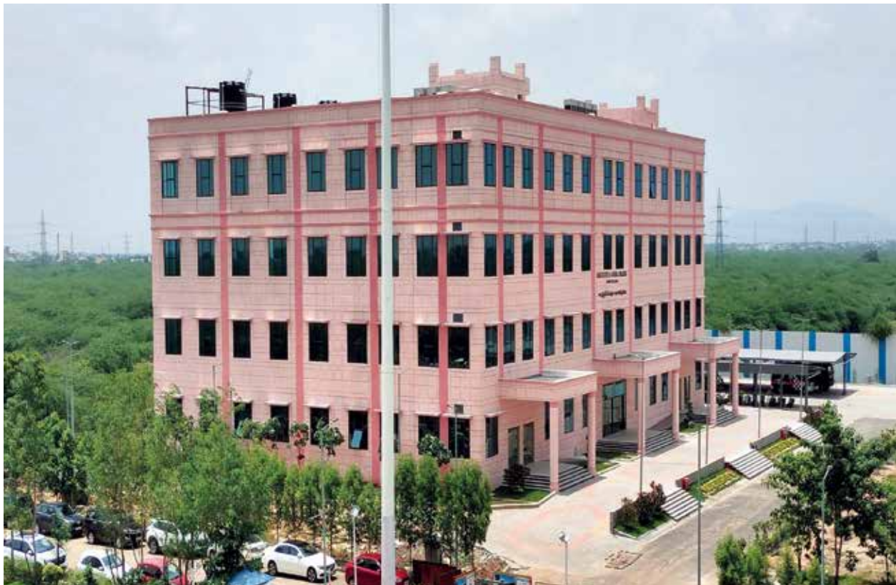
Lateral view of the Annexe Building of the High Court
