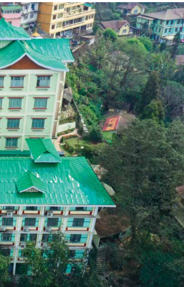
Aerial view of the High Court
