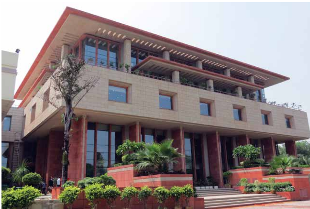
Front view of New Building of the High Court
