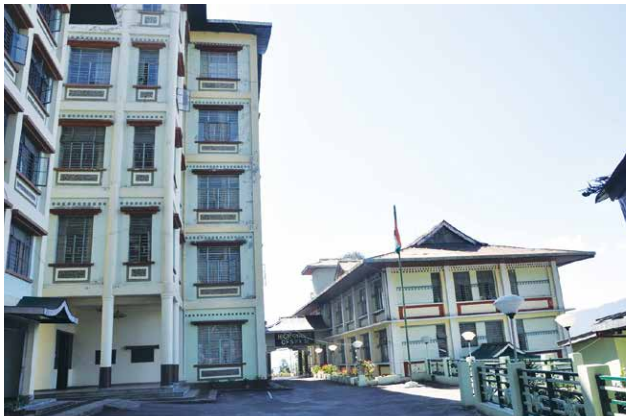
View of the High Court
