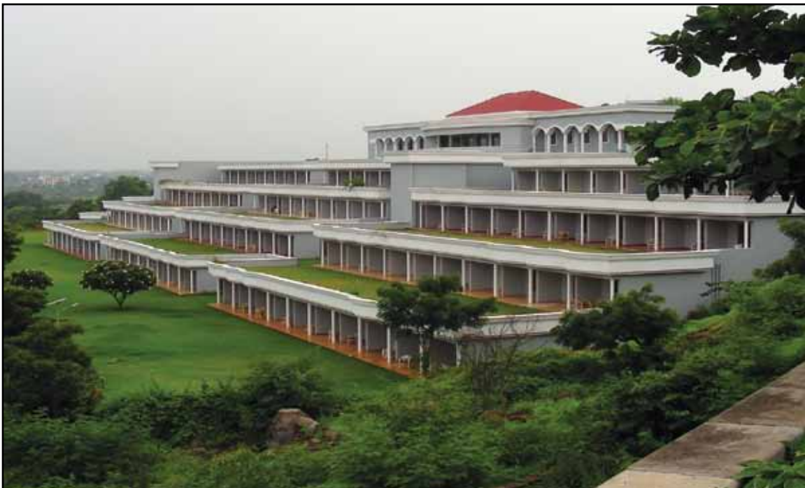
Elevated view of the National Judicial Academy at Bhopal
