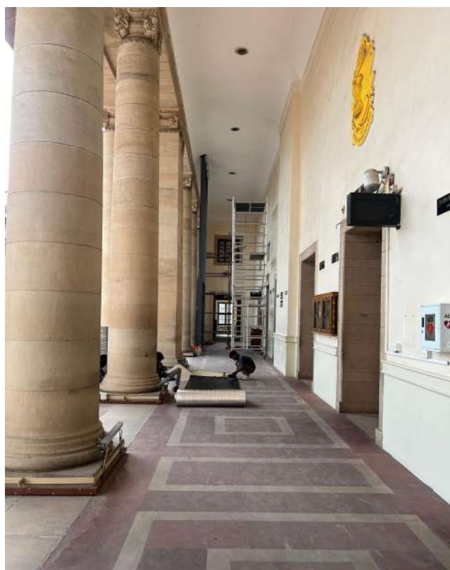
Ongoing repairs at Supreme Court during summer vacation
